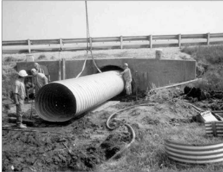
■ Figure 12.3 Typical slip lining installation with a pipe arch shape to suit existing cross-section.
