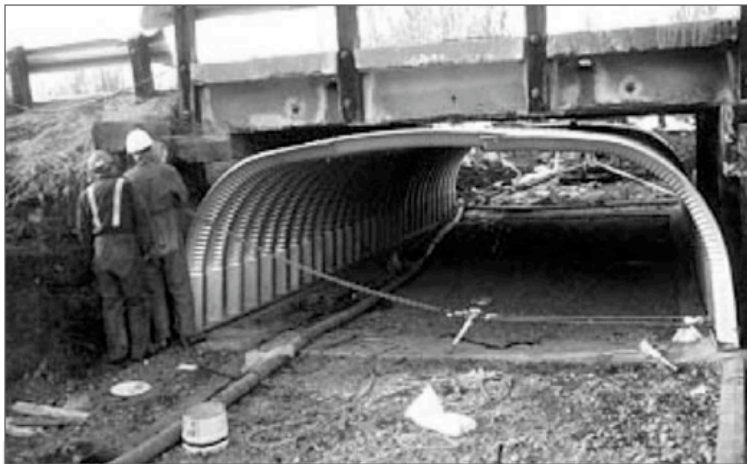
■ Figure 12.7 Deep corrugated box culvert lining a falling bridge. Note the dozer pulling the corrugated box culvert into position.
