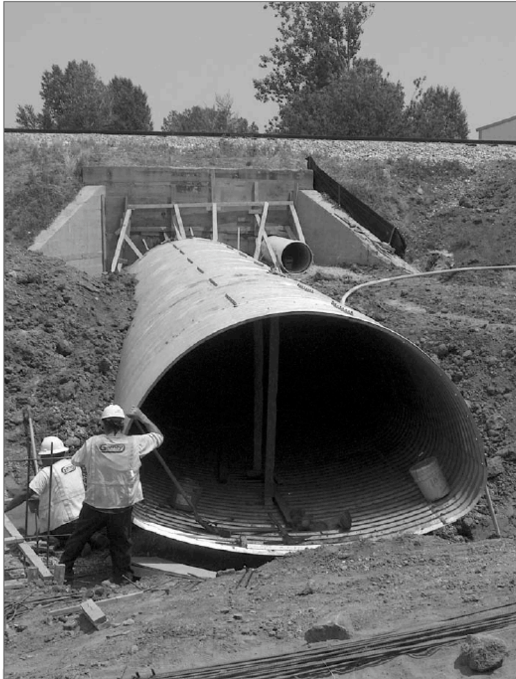
■ Rehabilitation & extended concrete box.
